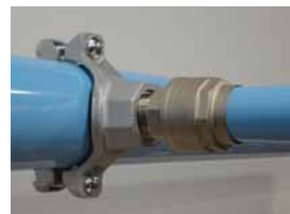
Attach Quick-Lock piping to fitting
